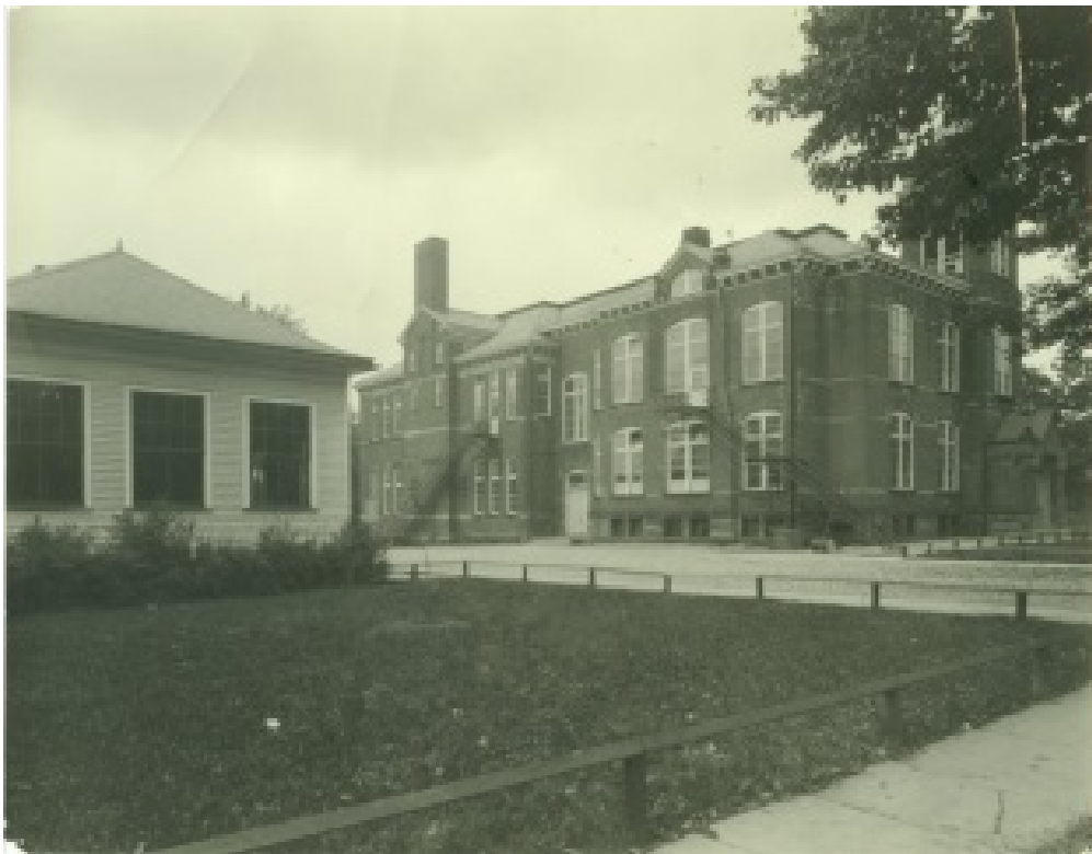
1909 1 st , 2 nd grade addition (Left of 1885 School Building) on Philomethian Street
