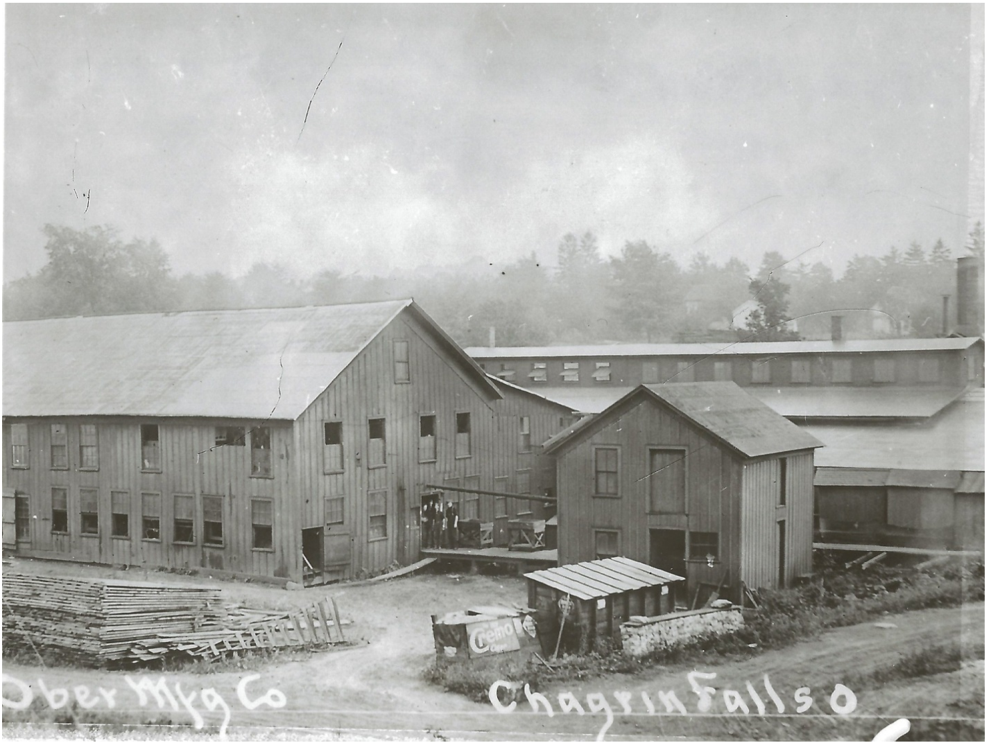
Manufacturing Buildings – view looking southwest from Bell Street
