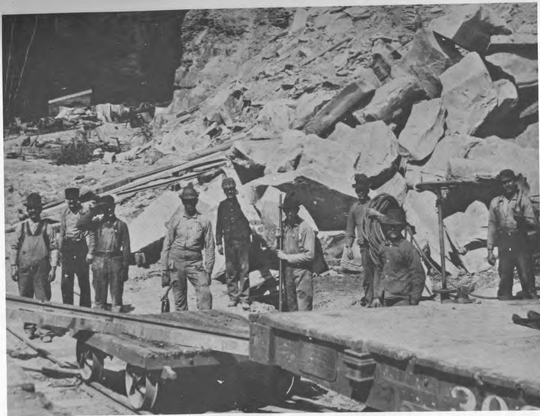
Stone quarry off Solon Road on the east bank of the Aurora branch. A narrow gauge railroad carried the stone to Solon to the Erie Railroad. Henry Church got some of the stone for his sculptures from this quarry.
