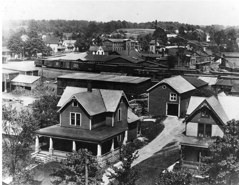
Figure 3. View of the steam railway yard from the top of the Philomethian Street School.
